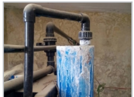
Scaling on RO Membrane
