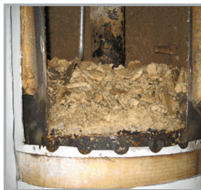
Water heater opened up revealing heavy scale accumulation
