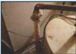
Scaling outside the Pipe
