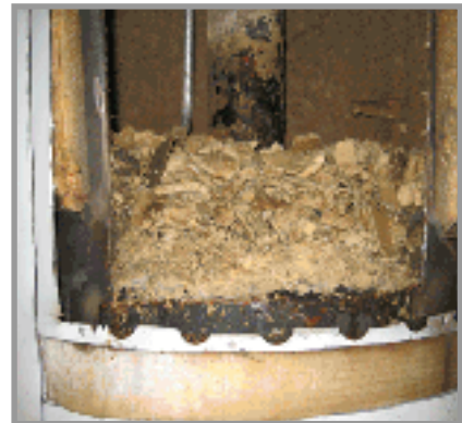
Water heater opened up revealing heavy scale accumulation
