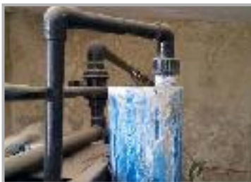
Scaling on RO Membrane
