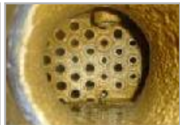
Scaling in Compressor
