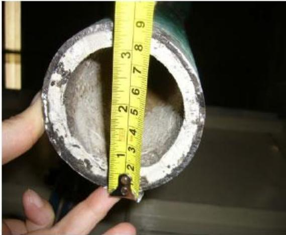
5. The scale thickness are over 10,000 microns inside the pipes.
