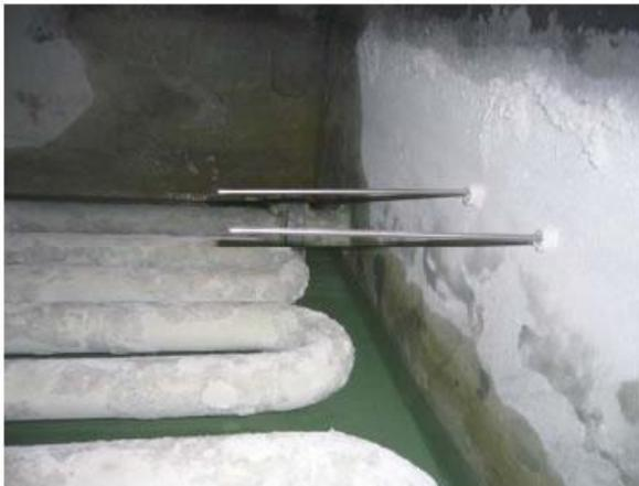
3. The objective of installation Magstream P-75 is preventive of sludge on the Heat Exchanger and control the Temperature consistence.
