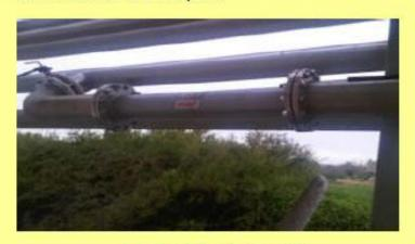
MagCAT installed at Alier Papel.. no electricity No moving parts
