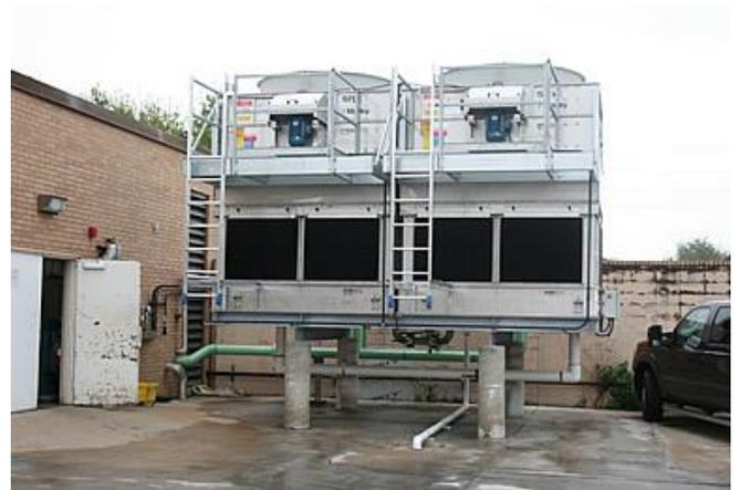
**The Challenge:** Walker Station was struggling with heavy scaling issues in their HVAC cooling tower / chiller system despite the use of scale prevention chemicals. The system was so heavily scaled and corroded that following a system assessment it was determined that replacement of the system would be more economical than repair.
